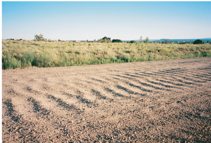
FIGURE 214 Road corrugations (courtesy David Mays).
